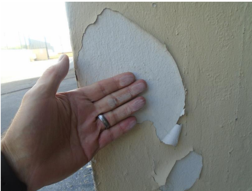
Example view of paint loss of adhesion-chalkiness under substrate-poor surface prep
