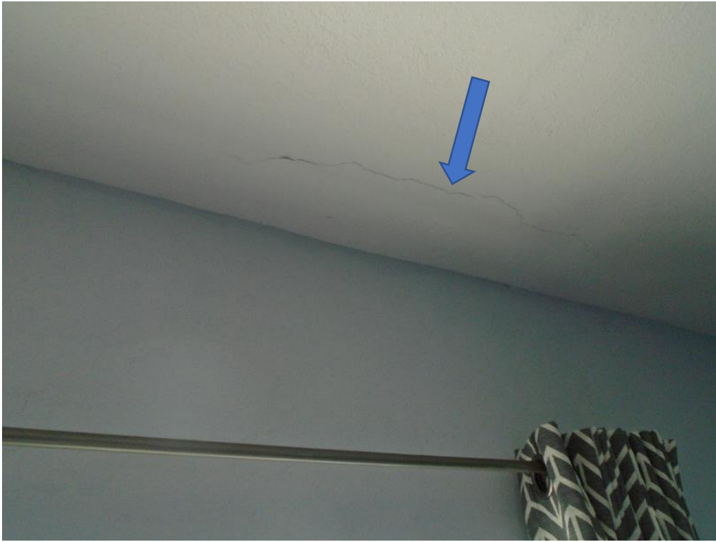
Example view Interior Ceiling Concrete spalling due to reinforcing steel corrosion
