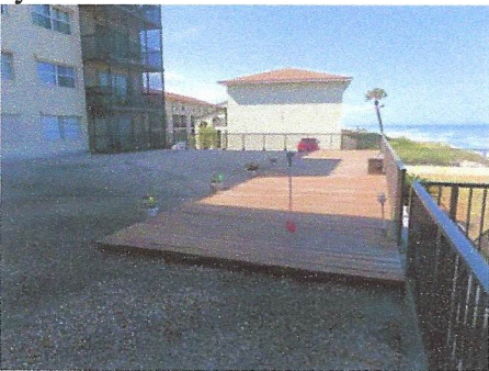
General view of tar & gravel roofing system on lower section
