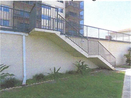
View of east side stairway from rear deck
