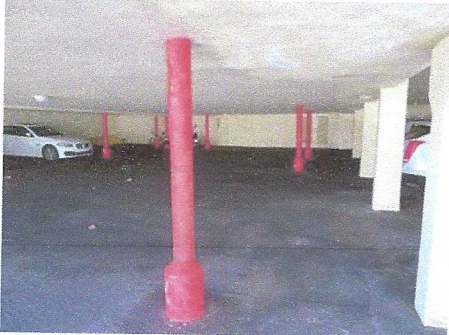
General view of typical north covered parking area columns
