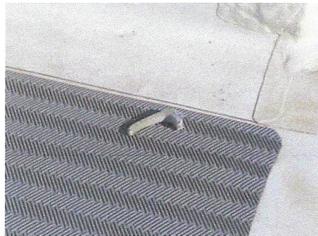
View of latch on roof deck
