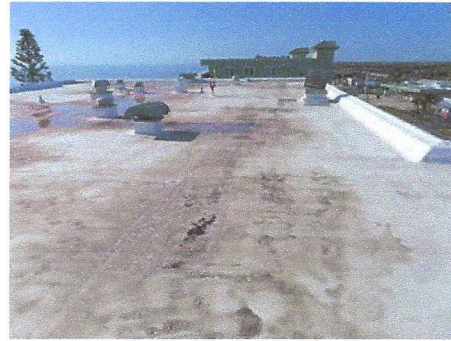
General view of single-ply roofing system on main section
