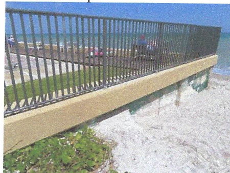
General view of seawall south elevation
