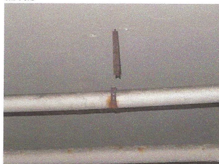
Closer view of piping supports which have rusted away in covered parking areas
