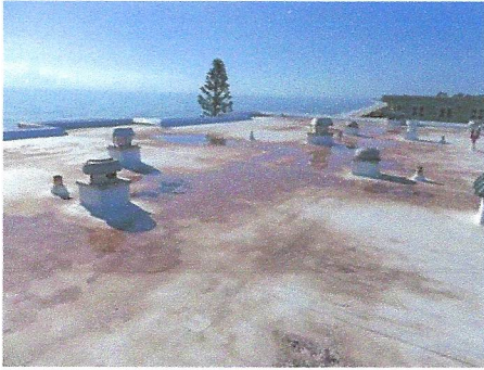
General view of single-ply roofing system on main section
