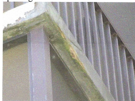
View of typical cracks on balcony corners which should be opened and/or sounded for spalling
