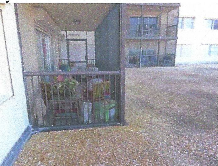
General view of tar & gravel roofing system on lower section
