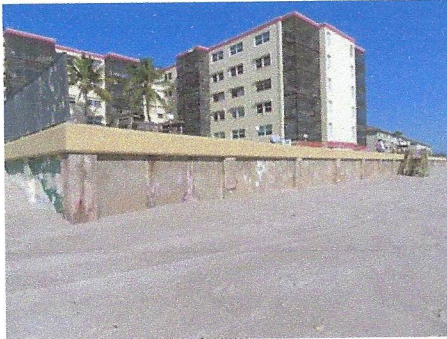
General view of seawall east elevation
