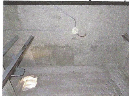
View of top of elevator hoistway
