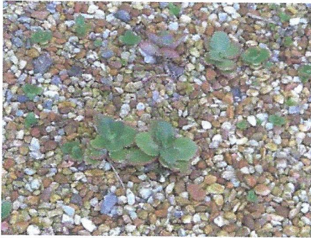
View of typical vegetation growth on the lower roof surfaces
