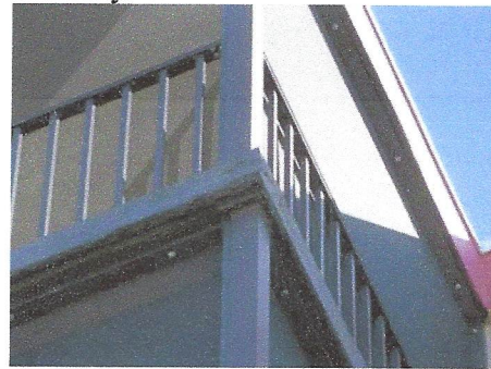
View of typical cracks on balcony corners which should be opened and/or sounded for spalling
