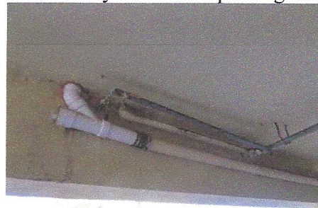
Closer view of piping supports which have rusted away in covered parking areas
